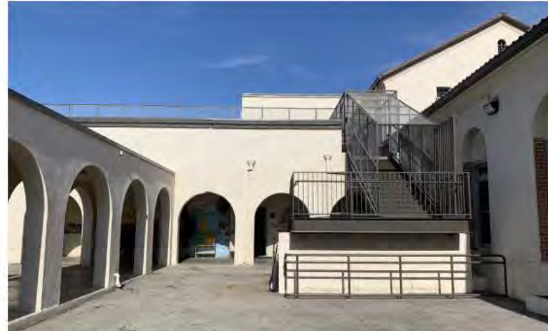
EXISTING EXIT STAIR AT WEST END OF SOUTH WING
